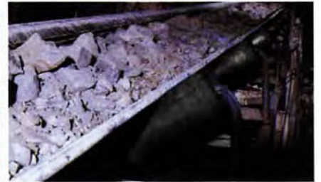
Limestone handling in cement plant
